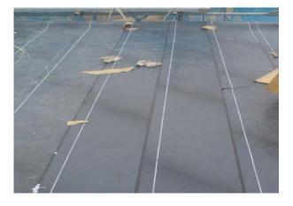
TamSeal 1500 is a cross laminated self-adhesive bitumen/ asphalt compound modified SBS preformed waterproof membrane comprising with high performance HDPE carrier film. TamSeal 1500 is suitable to use for above and below ground, on vertical or horizontal surfaces where waterproofing is required. This product is formulated for easy installation as well as to achieve the final adhesion and finished in just a few minutes.
